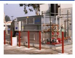
**Recold JC Evaporative Condenser**—Forceddraft, low profile design. G-235 galvanized steel factory assembled structure. Also available in 300 series stainless steel. Proven copper coil technology.
